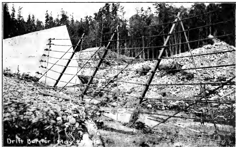
FIG. 9.—INTERMEDIATE WORK, DRIFT BARRIER EXTENSION.
